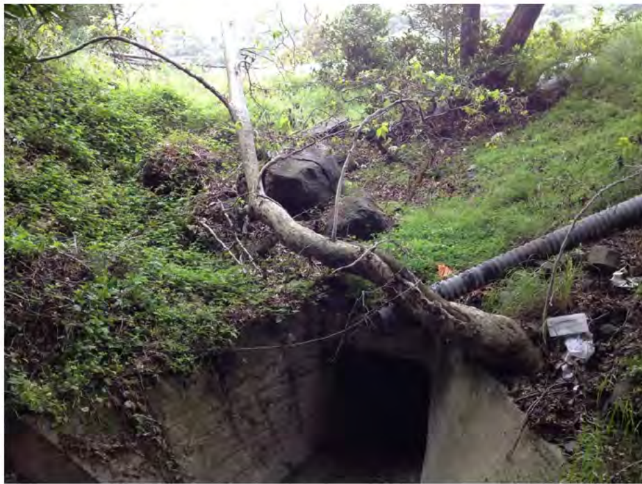
Figure 4: Ravine Culvert Inlet
