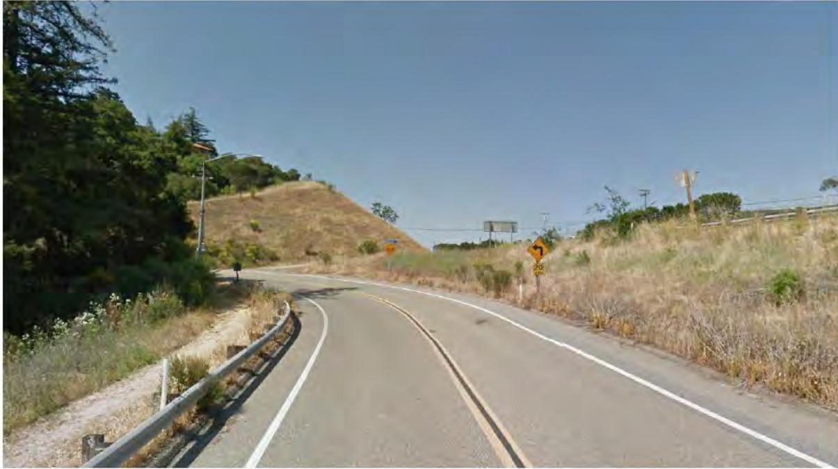
Potential undercrossing opening location – west side; about at “curve ahead” sign
