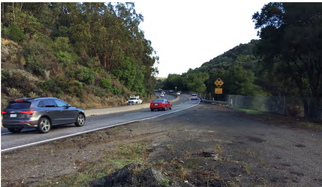
Photo 1: Alternatives 5/5a, looking north, View from the access ramp to northbound Highway 17
