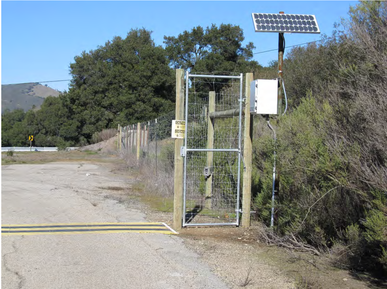
Photo 1: Example of "Electric Wildlife Mat", human access gate, directional fencing, and "jump out" feature Photo credit: 2012, Caltrans District 5, Nancy Siepel and Morgan Robertson
