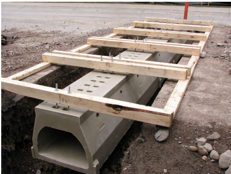
Herp (amphibian and reptile) crossing under construction - Waterton National Park, Alberta, Canada
