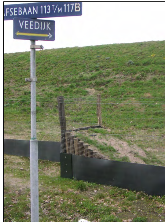
Example of fencing to direct small animals to a wildlife crossing in the Netherlands
