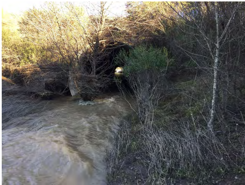
Figure 10: High water flowing through Lexington Culvert (January 13, 2017)
