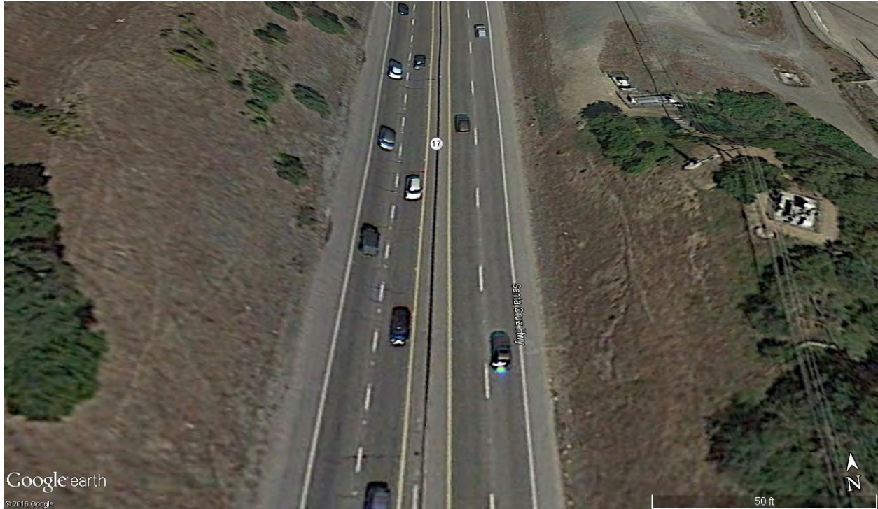
Potential overcrossing site looking north
