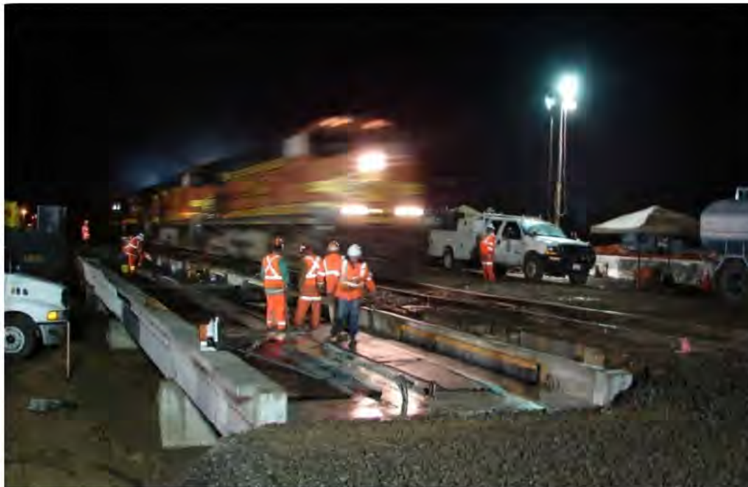
Figure 8: Pile Supported Precast Slab Bridge Construction
