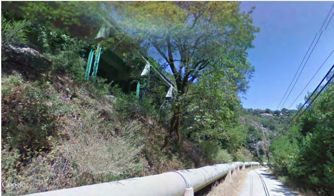
Figure 29: Eliminated Alternative 6, looking north, View under viaduct from Los Gatos Creek Trail
