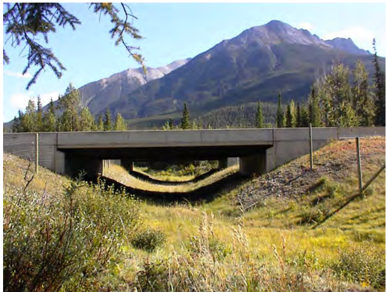
Example of wildlife undercrossing in Banff N.P. Alberta; Photo – Transwild Alliance.org
