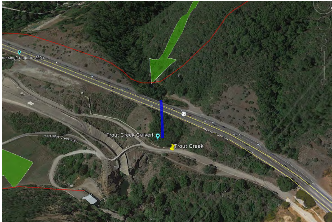
Trout Creek Canyon looking northwest – green arrows approximate wildlife path of travel (blue line is the existing culvert location - does not reflect the bend in the culvert)
