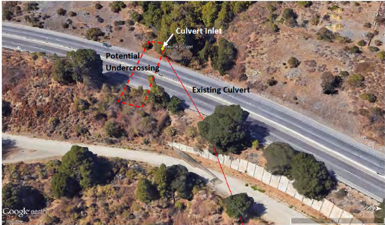
Figure 5: Ravine Culvert Wildlife Crossing Site View
