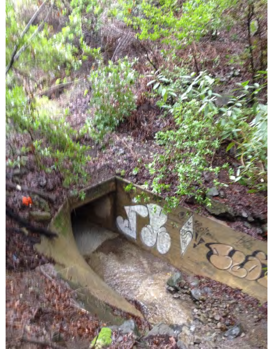
Existing culvert inlet on west side
