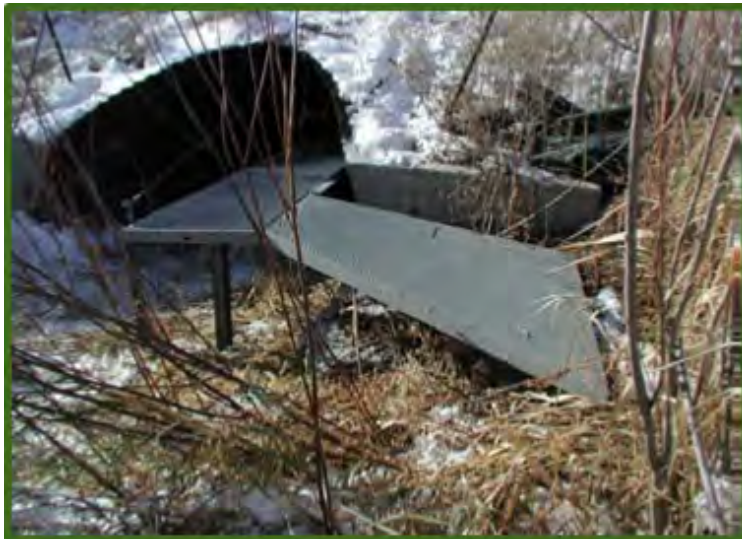
Figure 31: Example of raised catwalk inside culvert – Roscoe Steel and Culvert Co. and University of Montana’s “Critter Crossing”
