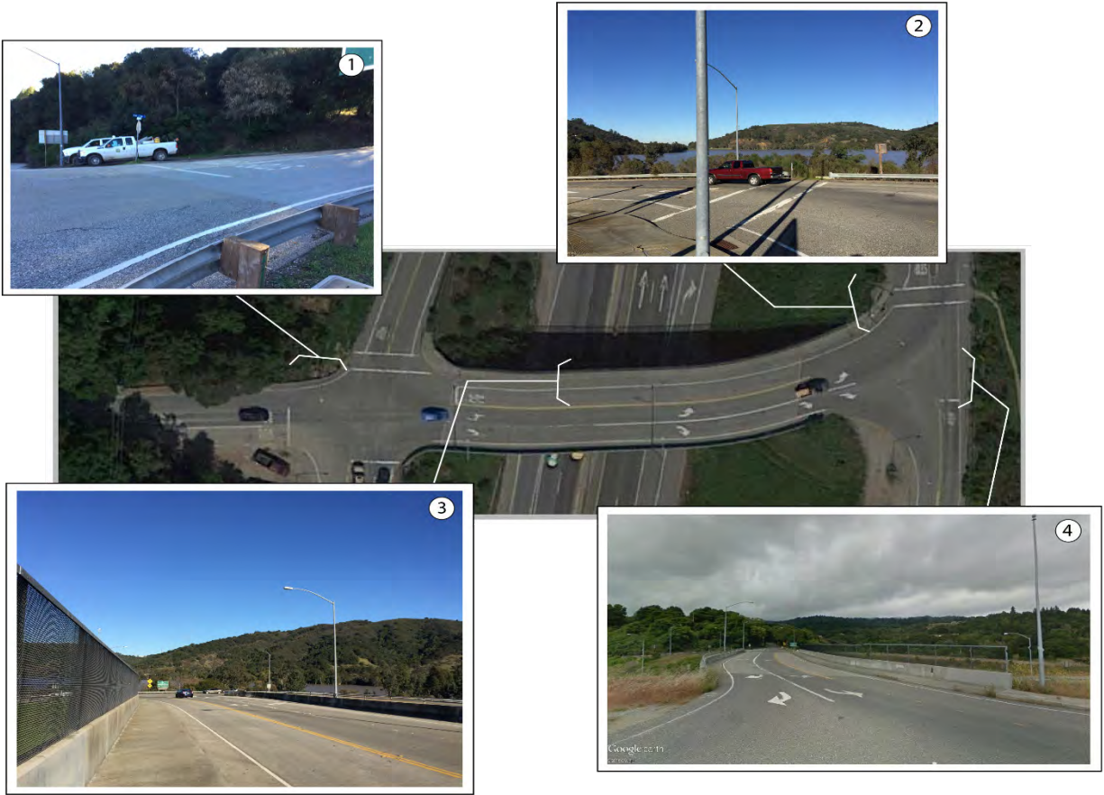
Figure 32: Bear Creek Road Overcrossing Existing Conditions
