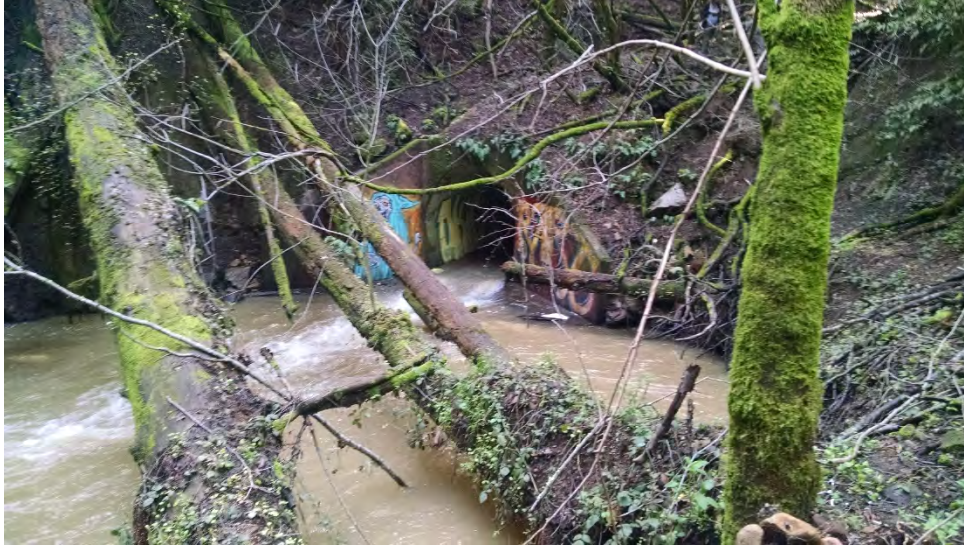
Photo 4: Aldercroft Culvert, Looking West During Wet Conditions
