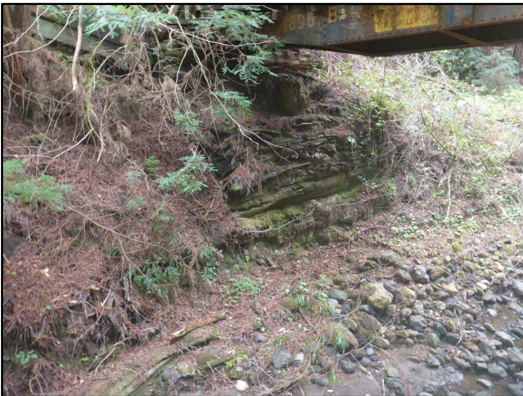
View bank under bridge at La Honda Creek on April 20. Bridge Site. Facing east.
