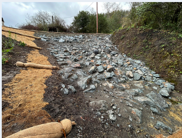
Completed construction of the engineered fill slope below Madonna Dam. Purisima Creek Redwoods Open Space Preserve (Sean Yao)
