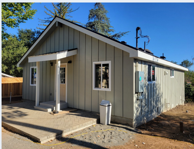
Structure improvements completed to serve as a new ranger residence. Sierra Azul Open Space Preserve (Paul Kvam)
