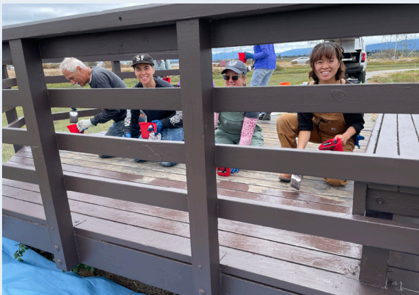
Volunteers from the Trails & Infrastructure Program repaint a popular viewing platform. Ravenswood Open Space Preserve (Judd Volino)
