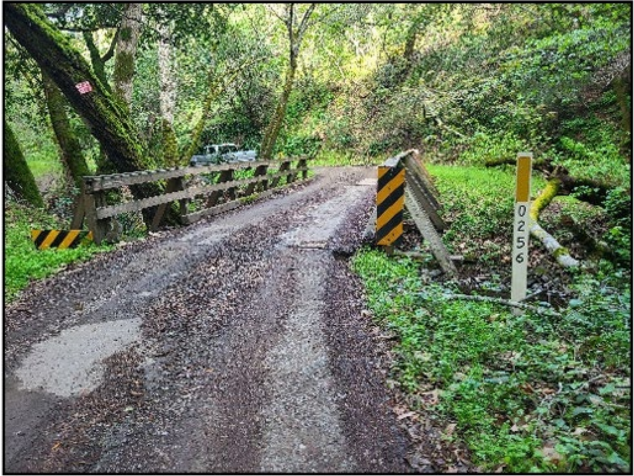
Example of existing vehicle bridges with timber guardrails and gravel road surface.
