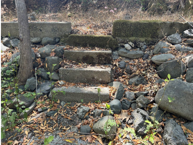
B3: Remnant concrete staircase.
