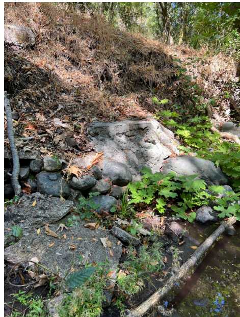
B20: Remnant concrete structure beside the creek.
