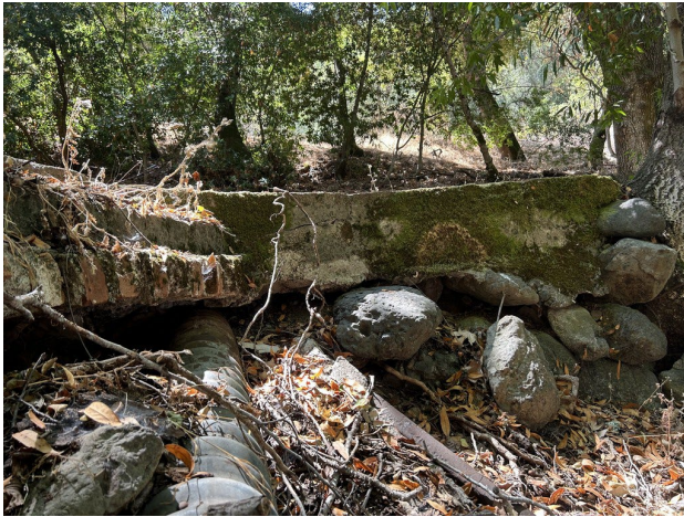
H5: Remnant concrete structure and associated materials.
