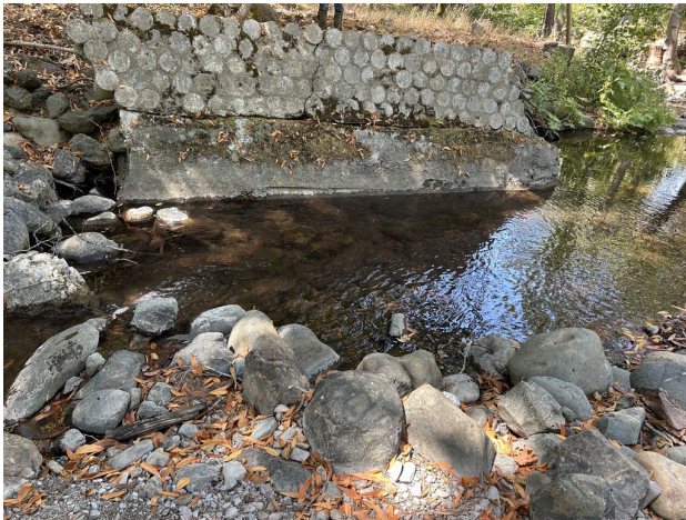
B7: Concrete retaining wall within creek channel.
