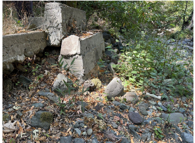
B3: Remnant concrete abutment beside the creek.
