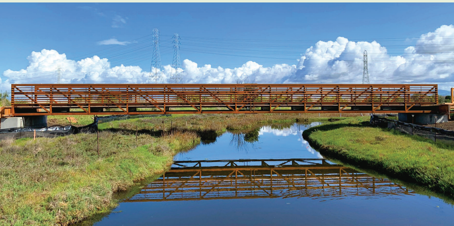
A recently installed bridge on the new San Francisco Bay Trail segment under construction
