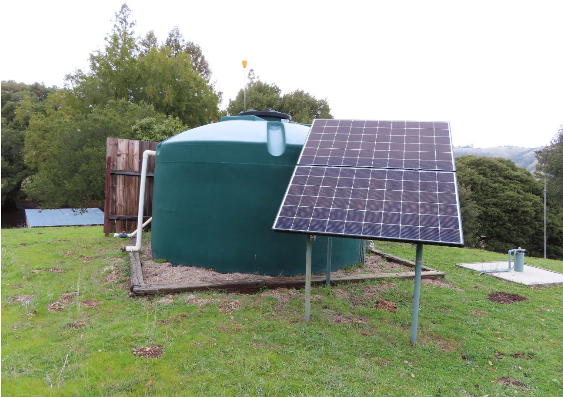
Water Tank and Solar Pump
