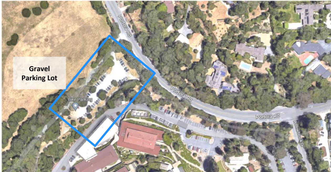
Figure 2 Parking Lot at Lower Windy Hill (Windy Hill Preserve)
