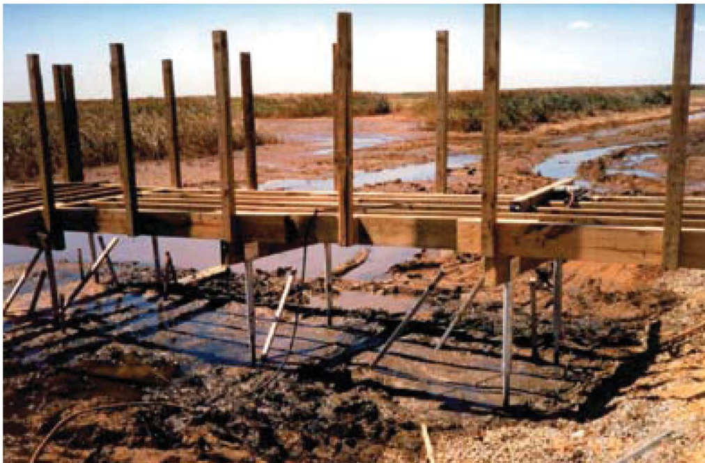
INSTALLATION OF SMALL-FOOTPRINT POSTS
